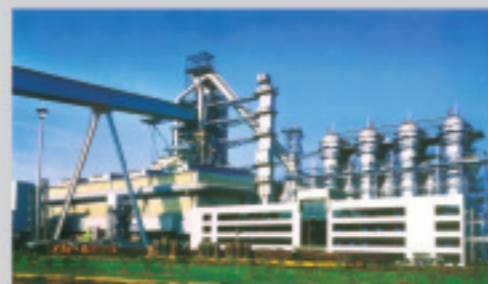
4350高炉 4350 blast furnace
