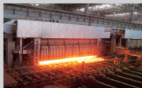
步进式加热炉 Walking beam reheating furnace
