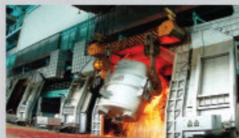
180吨顶底复吹转炉 180 ton top and bottom combined blown converter
