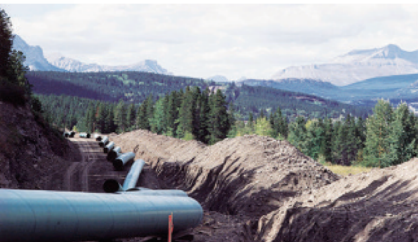
西气东输二线 Two pipelines from the west to the east
