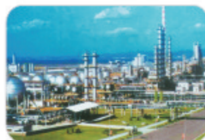
化工厂 Chemical plant
