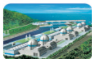
阳江核电站 Yangjiang nuclear power station
