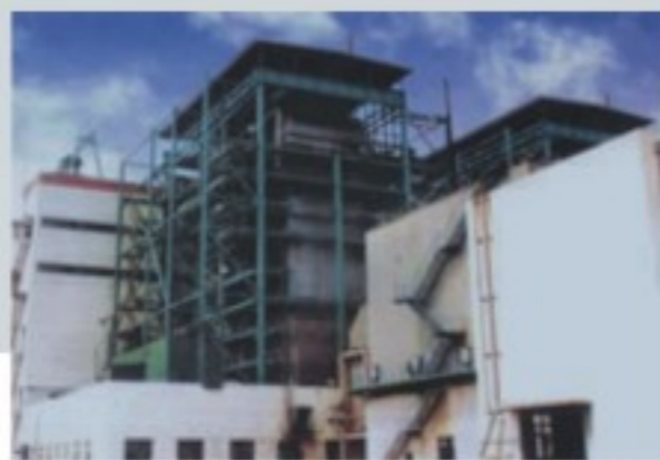
■ 流化床锅炉 Fluid Bed Boiler
